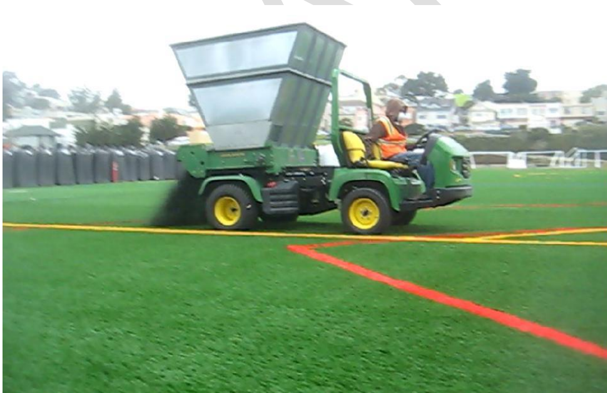
Figure A 9: Semi-mechanised application of infill
