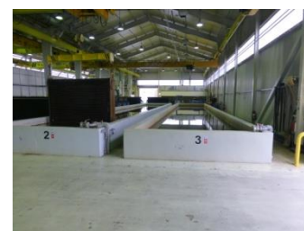
Storage Pits filled with water
