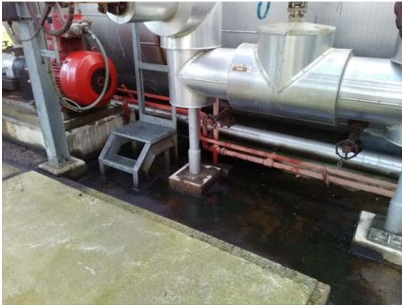
Figure 3. Air sample point in Site S-01
