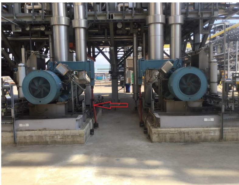
Figure 6. Air sample point in Site S-03
