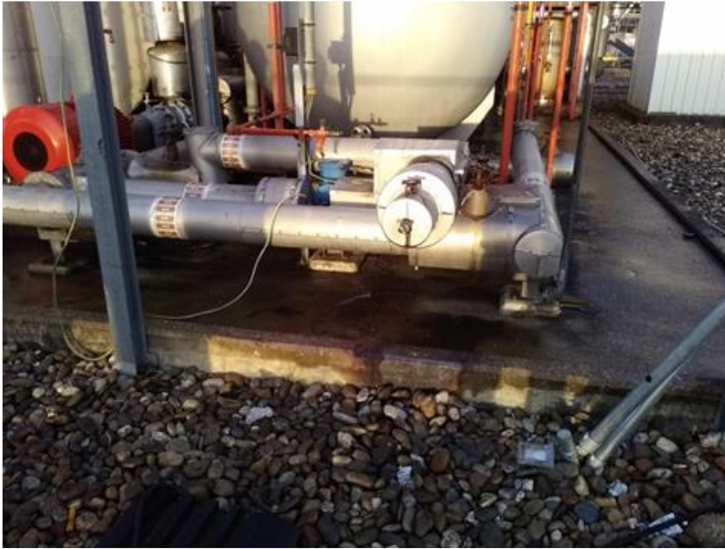
Figure 4. Soil sample point in Site S-01
