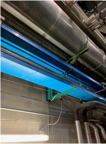
Figure 14. Air sample point in Site S-11 (transport pipes)
